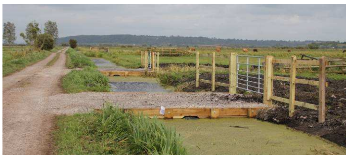
Timber pile and plank headwall culverts on North Drove
