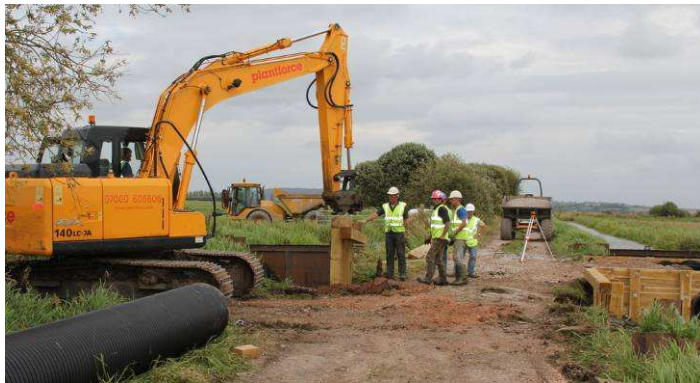
Construction of headwalls for replacement drove crossing
