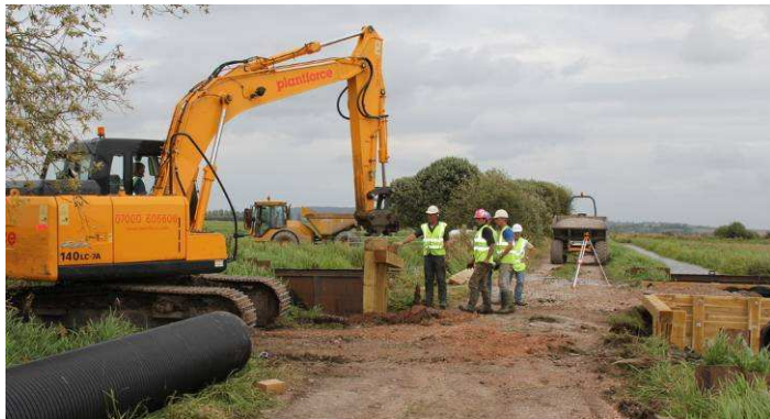
Construction of headwalls for replacement drove crossing
