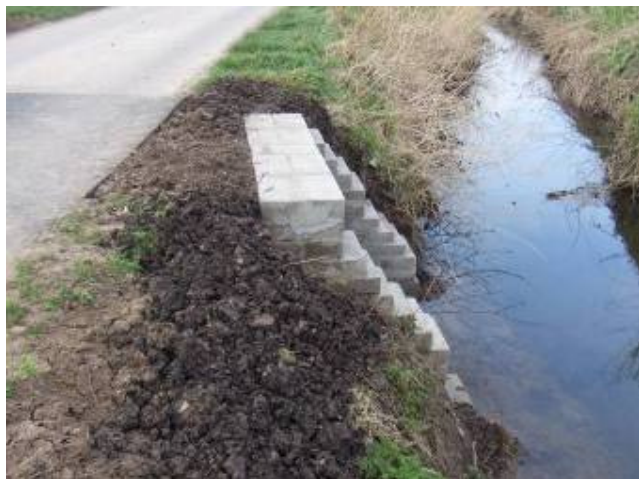
Replacement of road culvert at Helland
