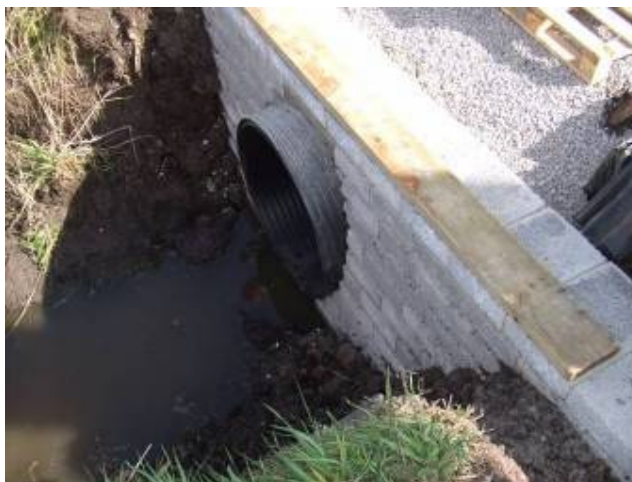
Concrete block head wall under construction
