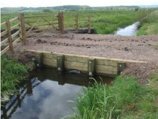
Timber pile and plank headwall - completed
