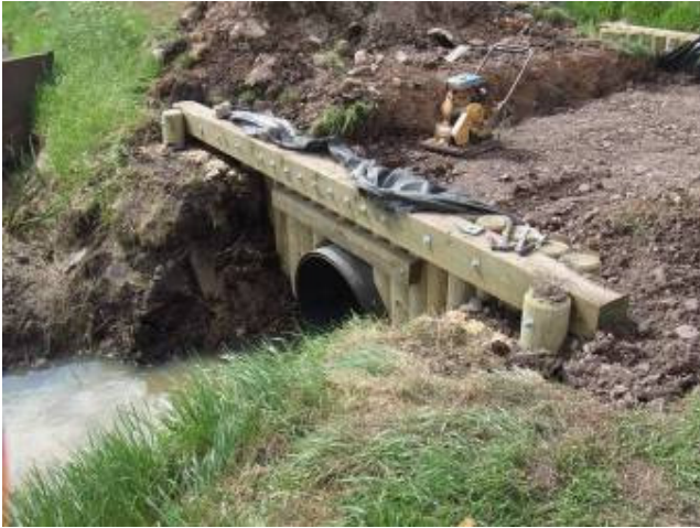
Timber post headwall under construction
