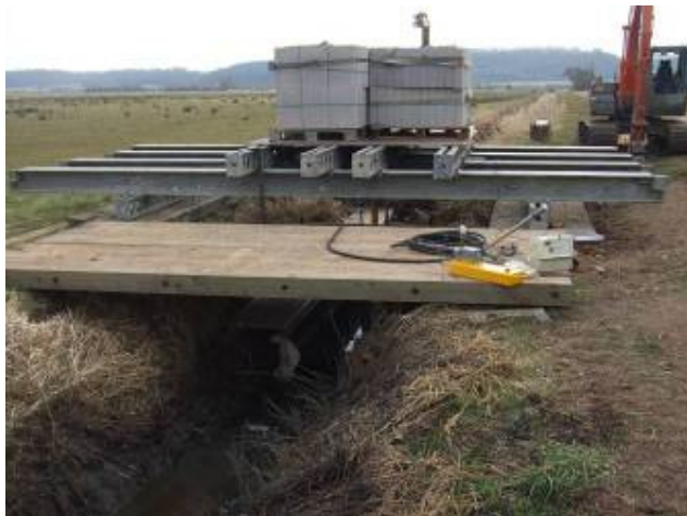
Timber pile load test
