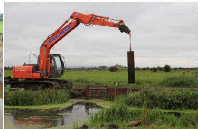
Decommissioning the raised water level area
