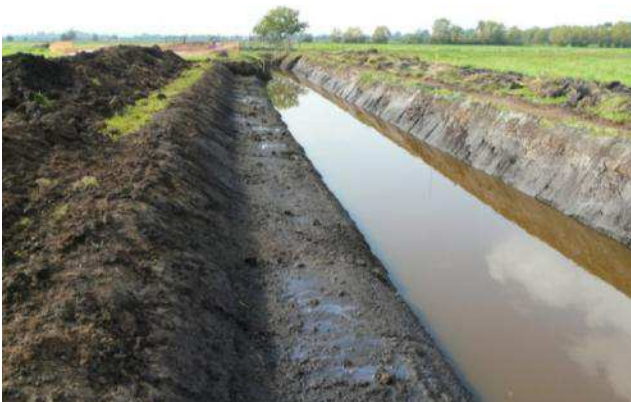
New inlet channel with two-stage profile
